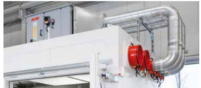
Fire protection flaps for ventilation system
