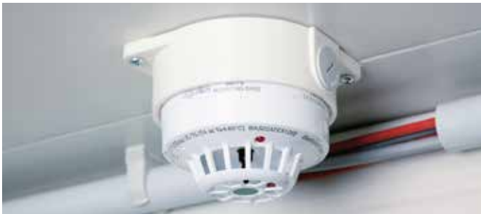
Industrial fire alarms
