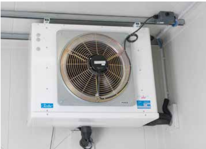
Split cooling unit (internal view)
