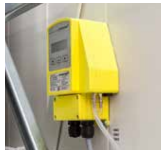
Air extraction monitoring
