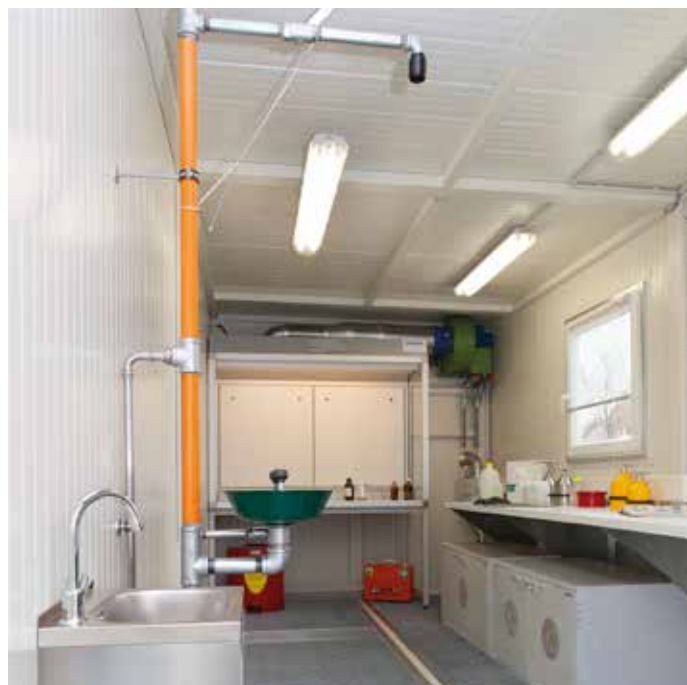
Sampling room with ventilation technology workplace and emergency shower. Additional safety is offered by fire-rated underbench cabinets for retained samples.
