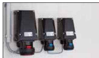
Sockets for connection of additional works equipment (230 V or 400 V, 50 Hz.)
