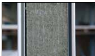
Fire protection panels in non-combustible A class material (mineral wool panels)
