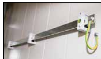
Earthing rails inside the technical room system
