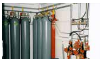
CO 2 extinguishing equipment
