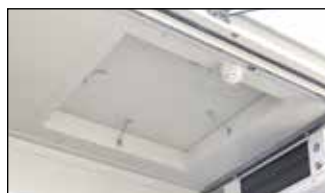
Roof pressure release panels
