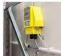
Air extraction monitoring for air exchange > 2.0/h
