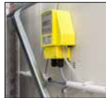
Air extraction monitoring for air exchange > 2.0/h
