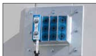
Fire protection insulation system for cable / pipe breakthrough points
