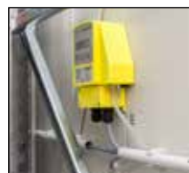
Air extraction monitoring for air exchange > 2.0/h
