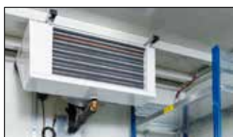
Climate control equipment for precision tempering in the inner room
