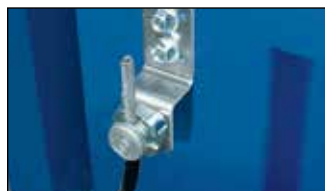
Earthing point for customer earthing of the technical room system
