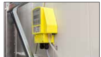
Air extraction monitoring for air exchange > 2.0/h
