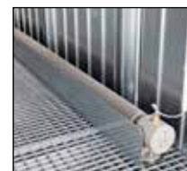
Finned tube heater with impact protection
