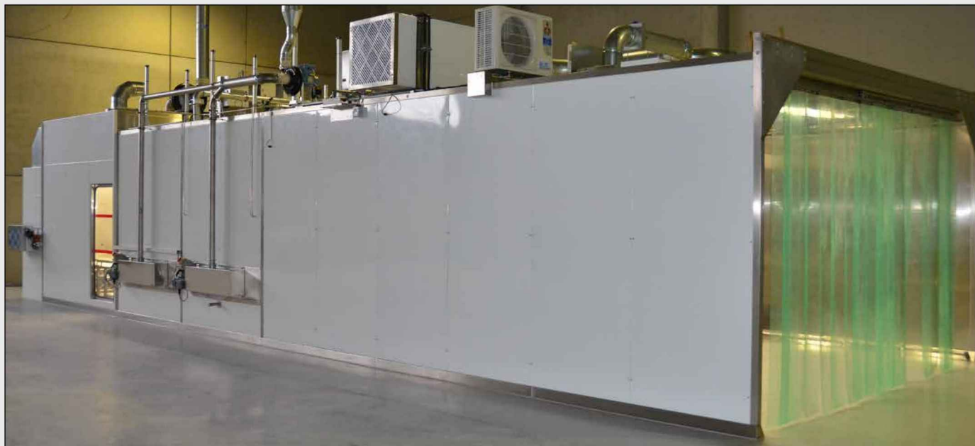
Sampling equipment with material pass-through, lift, personnel air lock, material air lock with automatic conveyor belts and sampling booth – including automatic IPA disinfection area
