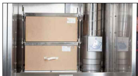
Filter cells in the rear wall of a free workstation
