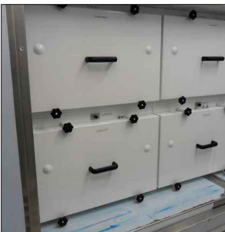
Filter housing for contamination-free filter replacement
