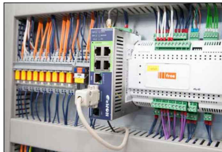
Connection of monitoring sensors to client's process control systems
