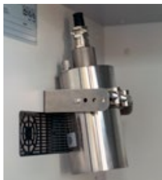
Electronic fire suppression system
